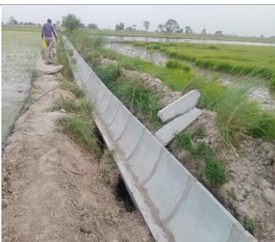
Figure-4.76: Slope issue at Watercourse In Kalianwala of watercourse no18715/R
