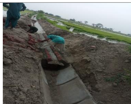
Figure-4.79: Work under process of watercourse no18715/R
