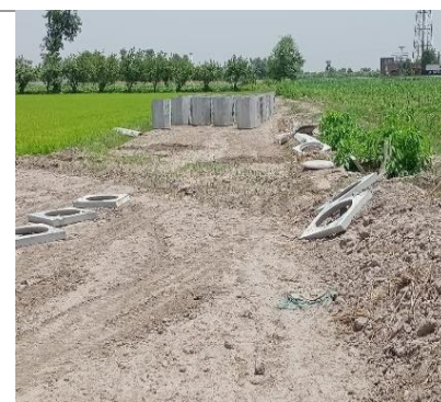
Figure-4.73: Improper placement of Segments & Naccas on watercourse no 21600-R
