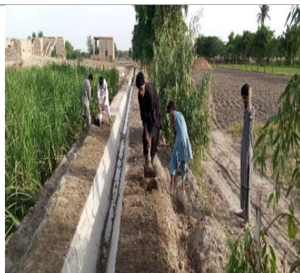
Figure-4.101: Backfilling process in progress at water course 94934 L
