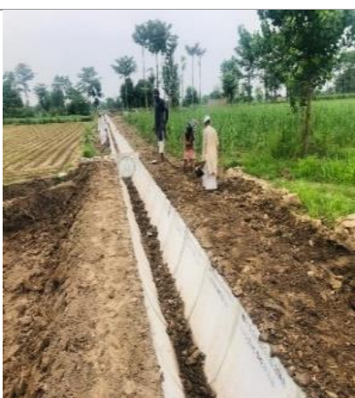
Figure-4.68: Proper back filling of watercourse 11430/R
